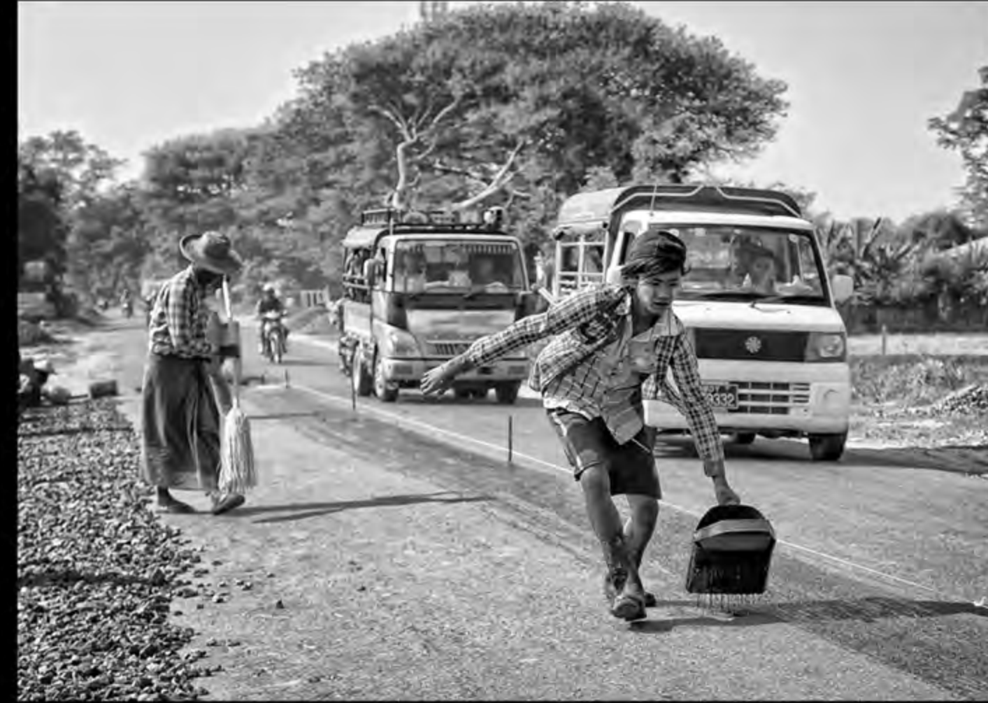
Wing Chung Kenneth Leung EPSA Hong Kong Road Repair BW
