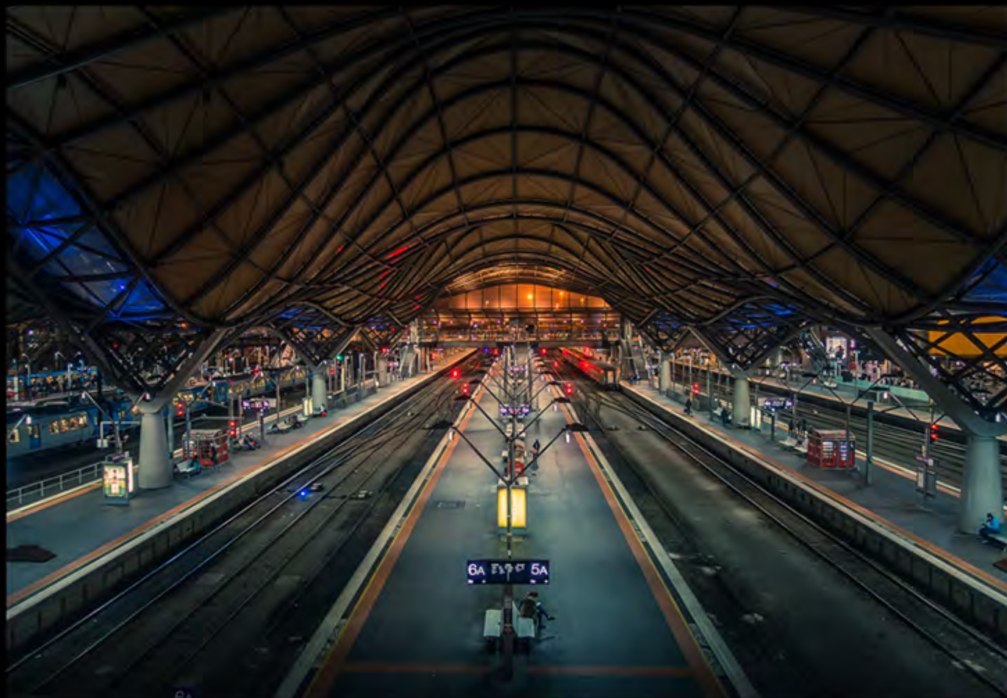
Trace O'Rourke Australia Southern Cross Station
