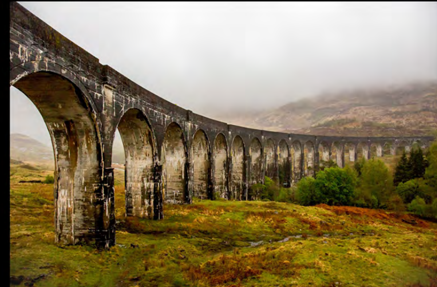
Martin Newland Australia Viaduct at Glenfinnen - Scotland
