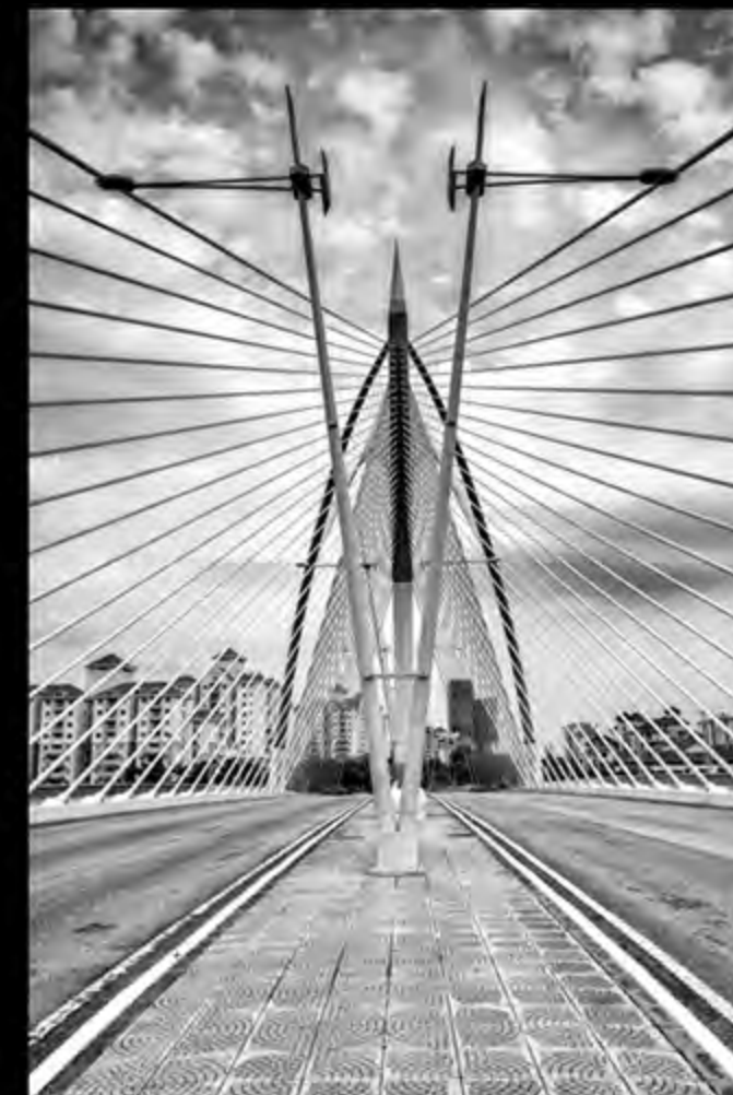
Vicki Moritz EFIAP/g MPSA GMAPS Australia Wawason Bridge Putrajaya
